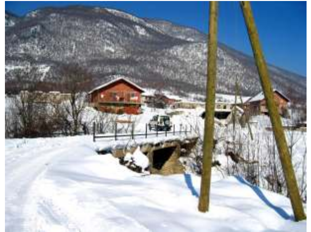
IOM Trust Fond infrastructure project in the minority village of Siga-Peja/Pec Municipality
