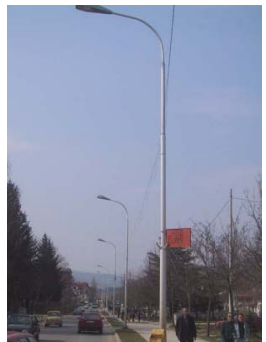
Kamenica Street Light Upgrade
