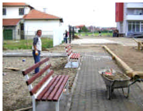
Construction work at Roma Mahalla in Mitrovicë/ Mitrovica
